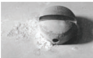
Figure 2. Galvanic Corrosion between a Stainless Steel Screw and Aluminum. A Cathodic Material for Fasteners is Preferred.[2].
