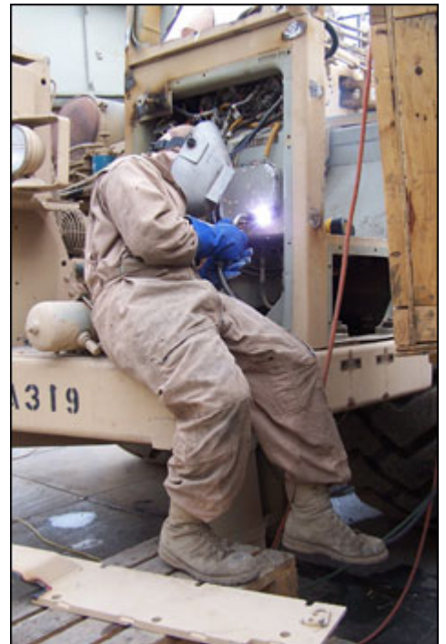
Spc. O'Neil Gaynor, a welder with the 16th Engineer Brigade's Headquarters Support Company, 62nd Engineer Battalion focuses his attention and torch on the final preparation of a scraper before welding on new armor at the brigade's add-on-armor site. Gaynor works as part of the 12-member crew who run Iraq's only Soldier-operated add-on-armor installation site. Sgt. 1st Class Tracy Ballog
