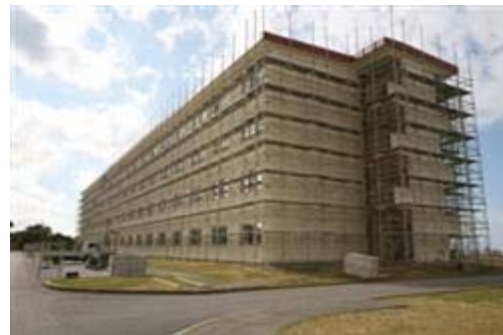
Scaffolding surrounds building 470, a barracks on Camp Foster. The Facilities Engineer Environmental Branch began recently testing an experimental paint in an effort to make government buildings more energy efficient. (Photo by Lance Cpl. Thomas W. Provost)
